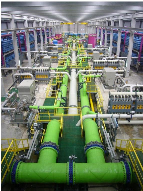
Figure 1: A reverse osmosis desalination plant. Most new desalination plants are of this type. (photo: James Grellier)
