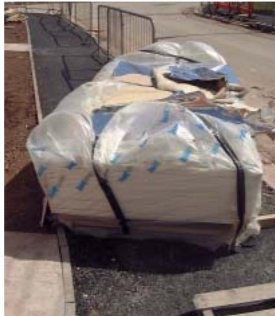
Figure 11: Boards stored in a central location.
